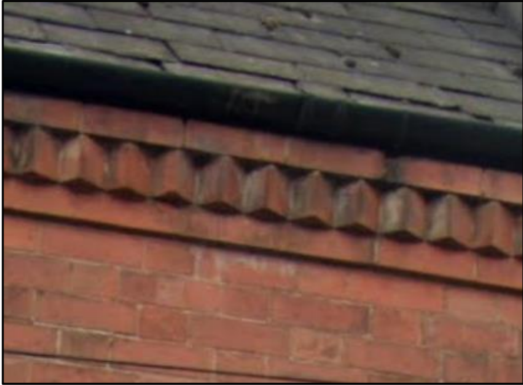
Photo: Dog Tooth Eaves or Cogging
