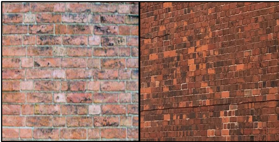
Photo: Flemish Bond left and English Bond right
