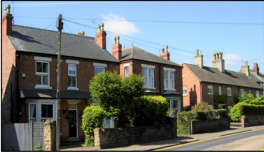
Photo: 90 - 92 Main Road (left) and 86, 88 Main Road, Grade II Listed cottages (right)
