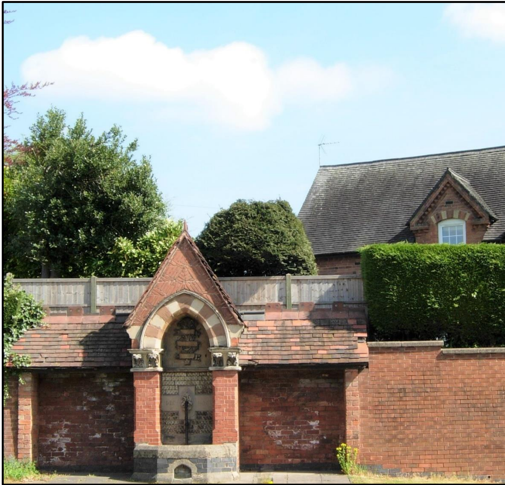
Photo of the Fountain with Fountain Cottage behind note polychromatic brick work on window lintels matches the stone arch on the Fountain (bottom).
