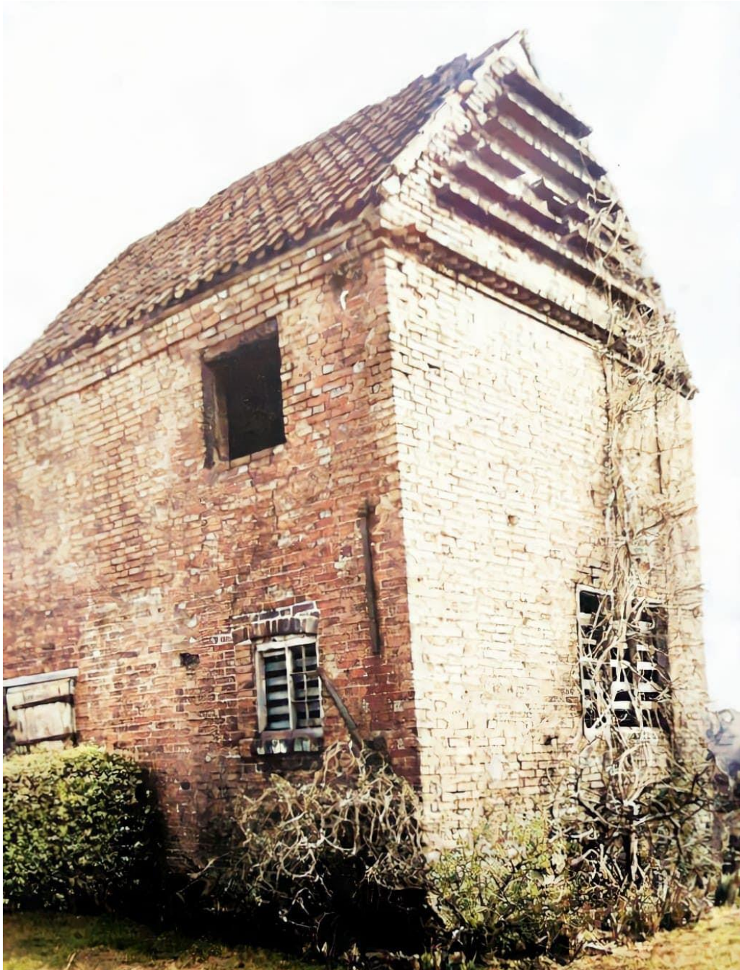
Dovecote now demolished. Photo with kind permission of the Gedling Village Local History and Preservation Society
