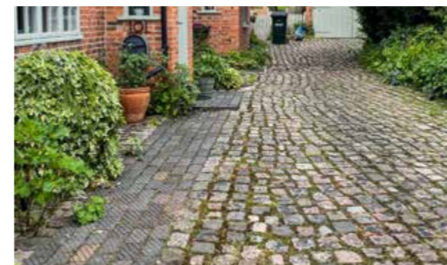
Locally distinctive surface materials include Staffordshire blue diamond pavers in Woodborough and granite setts. In Linby Limestone is used more extensively for paving slabs, setts and kerbs
