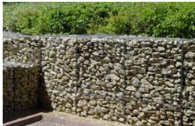
Example of a gabion retaining wall to manage changes in levels.
