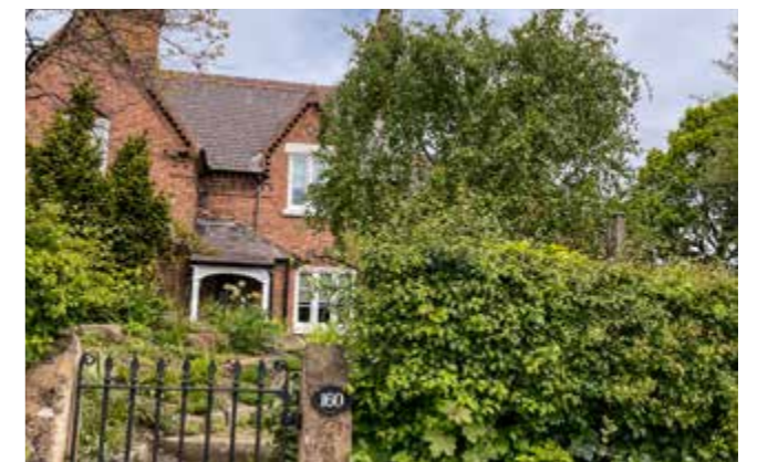
Calverton - large detached house on a generous plot contributing to a low density pattern
