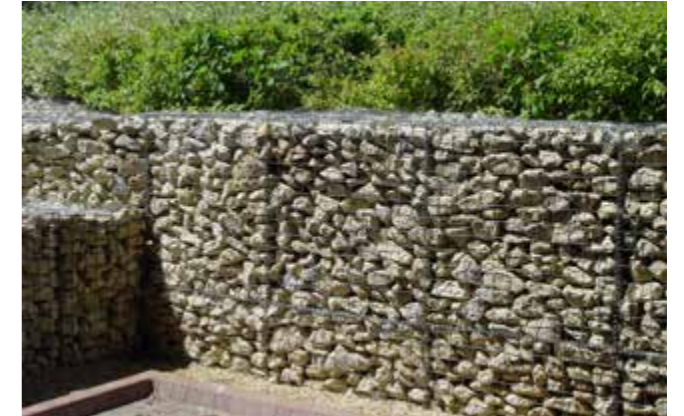
Example of a gabion retaining wall to manage changes in levels.
