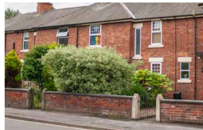
Continuous front boundary wall treatments in Bestwood, with distinctive gate pillars
