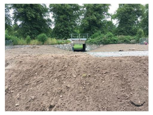
2.3 This image shows the newly constructed flood embankment at Tyne Green, Hexham.
