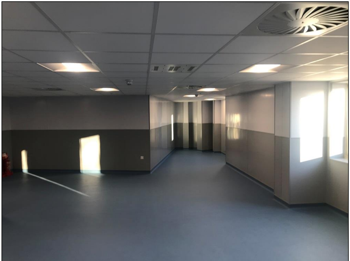
Vacant Future Locker & Canteen Area
