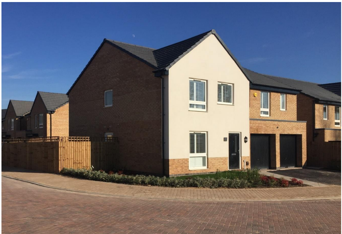
Photo new housing Gedling Colliery/Chase Farm
