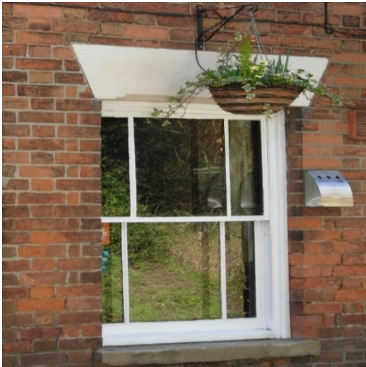
Photo cambered flat arch window at the Woodlark
