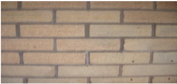
Photo of stretcher bond type brickwork
