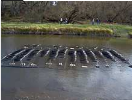
🏠 12-ton pond loop system being sunk to the bottom of a pond
