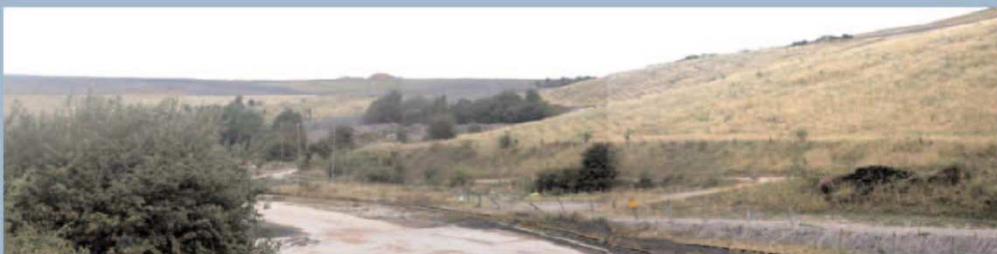
Site Photo - View looking north west along former railway line, where existing planting should be re-enforced to provide a buffer to the relief road.
