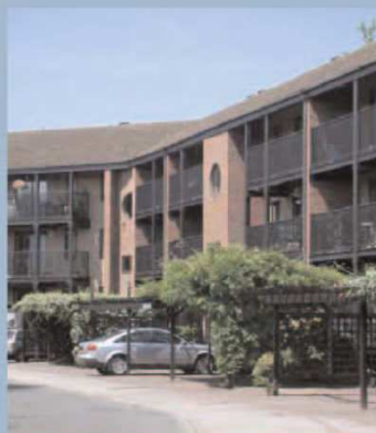
Contemporary and high density residential development in Nottingham.
