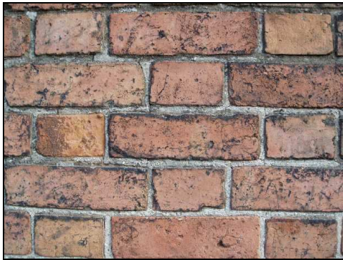
Flemish Bond brickwork
