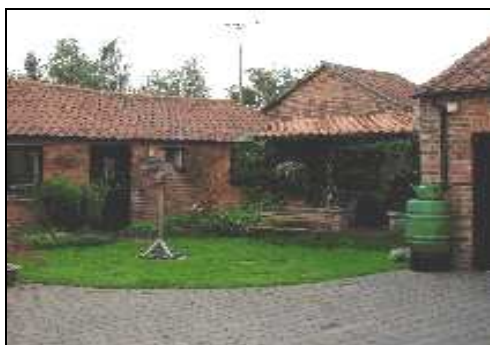
Outbuildings still in use
