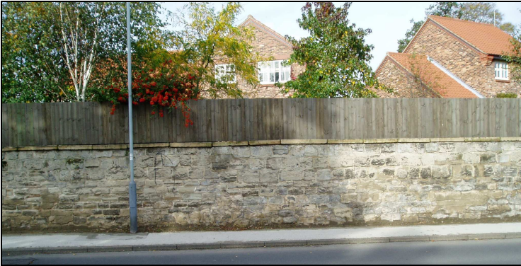
Old Hall Close boundary wall
